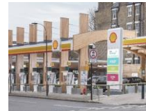
DC-Charging hubs @public
